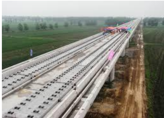
HSR construction in full swing
